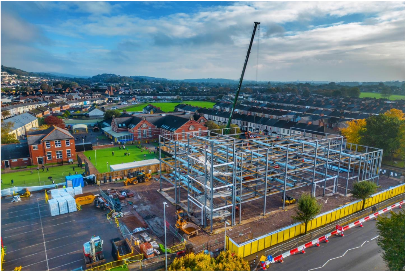
St Andrews School, City of Newport – Steel Frame being erected October 2023
